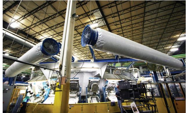
By placing 3” holes the length of the tubes, employees experience air movement without having to stand directly in front of a high velocity fan.
