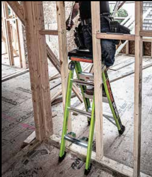
Fit Between Studs & Other Tight Workspaces
