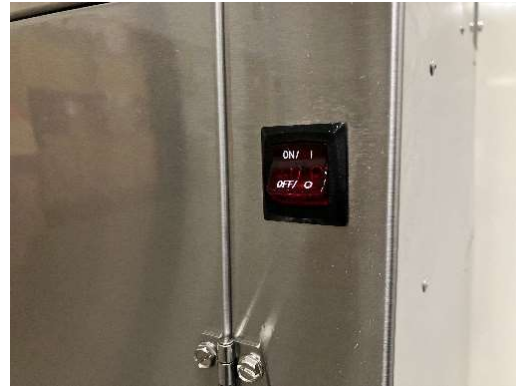
On/Off switch serves as a master switch for the internal receptacle for popcorn machine and warmer plugs
