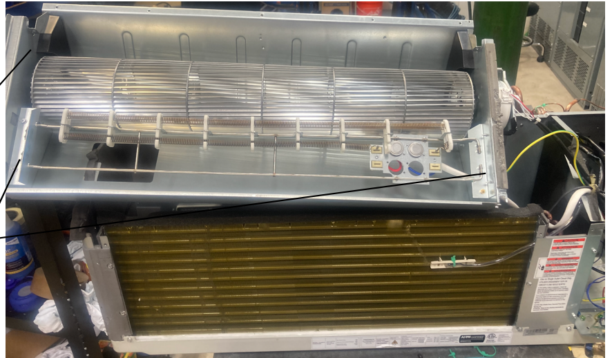
Figure 710 (Slide up Housing)
