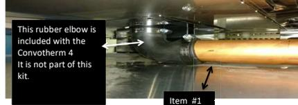
Pictured below is the drain line coming off the back of the oven utilizing 3 pcs. of item 1, two of item 5A, and one each of item 5C and item 5D (#5D Needs to be top elbow)
