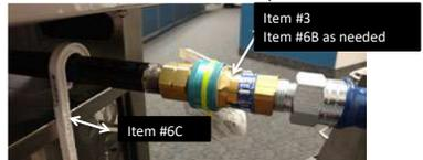
Pictured below are the incoming water lines on the side and bottom of the oven.
