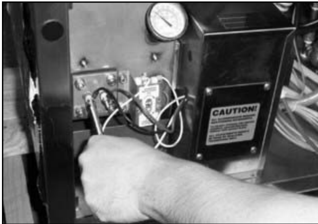
Removing the heater nuts.
