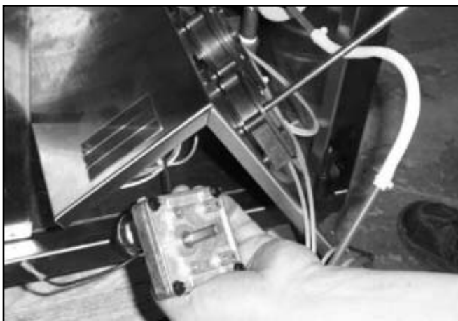
Removing the motor.
