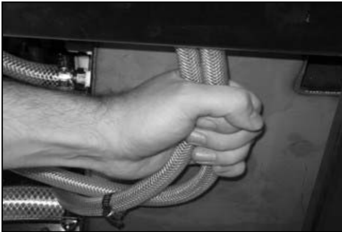
Pulling the discharge hose out.
