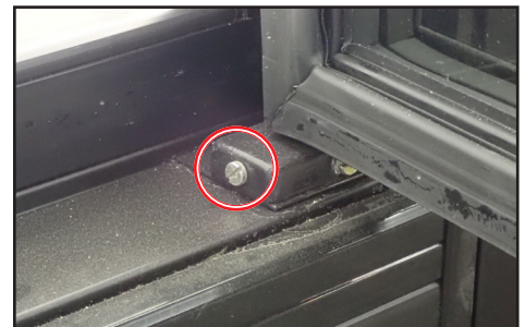
Fig. 25. Door alignment adjustment screw location. Clockwise turn: Adjust door handle-side down Counterclockwise turn: Adjust door handle-side up
