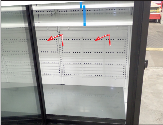
Fig. 1. Lift the interior backguard and pull it forward.
