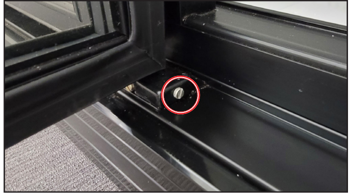
Fig. 2. Door alignment adjustment screw location. Clockwise turn: Adjust door handle-side down Counterclockwise turn: Adjust door handle-side up
