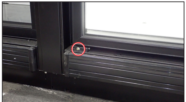
Fig. 6. Door tension adjustment screw location. Clockwise turn: Decrease door tension Counterclockwise turn: Increase door tension
