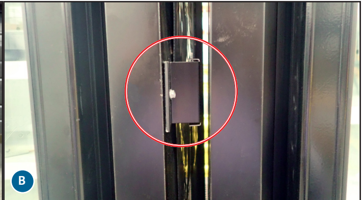
Fig. 10. Front bottom spacer touching the adjoining unit (A). Front middle spacers may not touch (B); this resolves during the leveling process.
