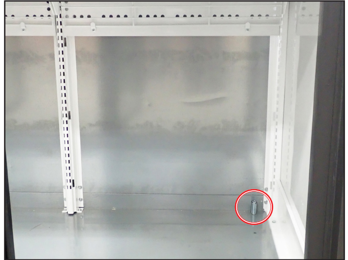
Fig. 2. Interior backguard removed to access rear leveling leg (circled).
