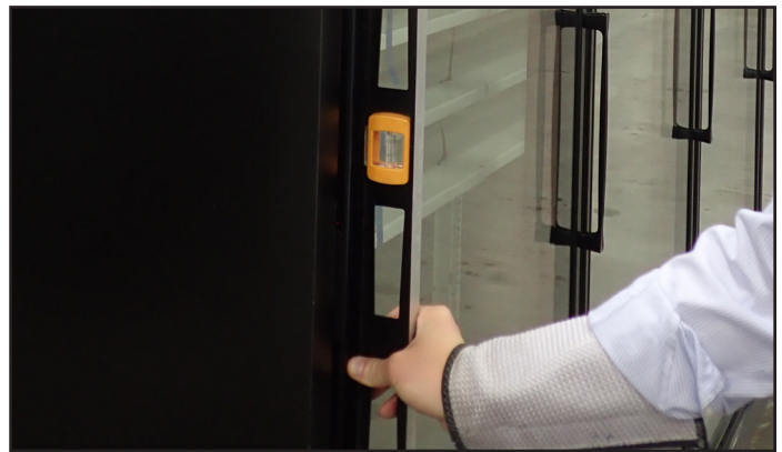
Fig. 6. Place the level on the door's hinged side. Level front-to-back.
