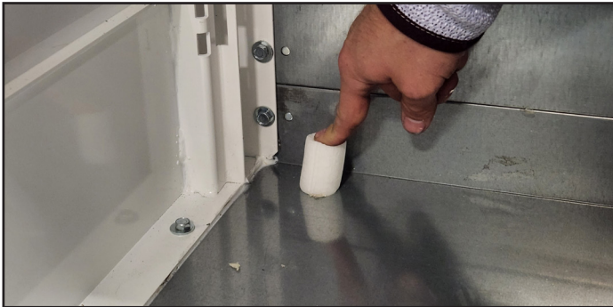
Fig. 1. Plug the leveling leg holes with foam.
