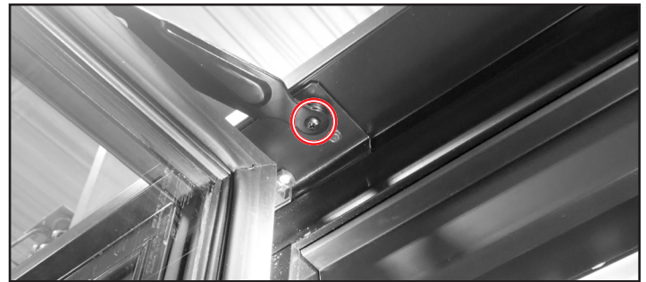
Fig. 1. Hold-open bracket screw location at the top of the door.
