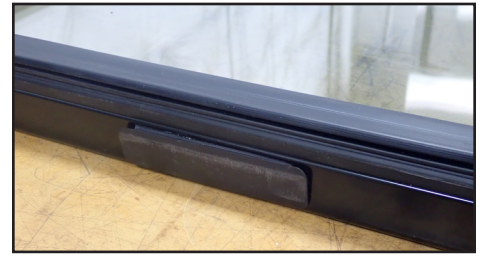
Fig. 6. Wire cover located in the hinge-side of the door in the center.
