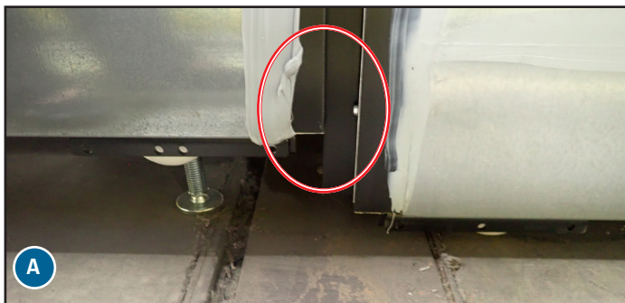
Fig. 11. Bottom of rear spacer touching the adjoining unit (A). The rest of the rear spacer may not touch (B); this resolves during the leveling process.
