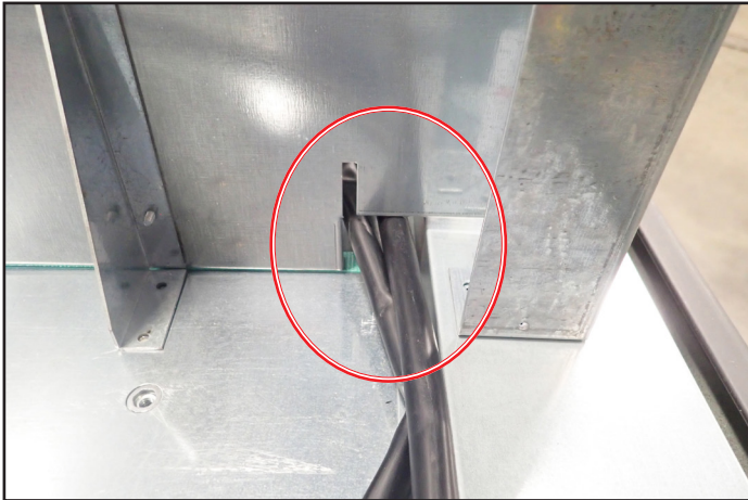
Fig. 3. Wires tucked into the air divider notch.
