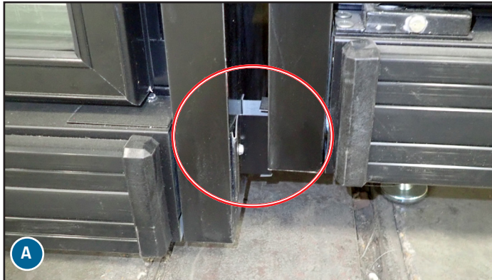
Fig. 10. Front bottom spacer touching the adjoining unit (A). Front middle spacers may not touch (B); this resolves during the leveling process.
