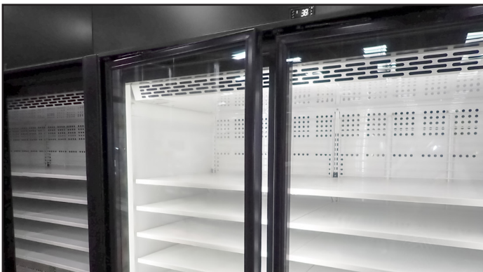
Fig. 5. Verify doors are self-closing when opened 2-3" (50.8-76.2 mm).
