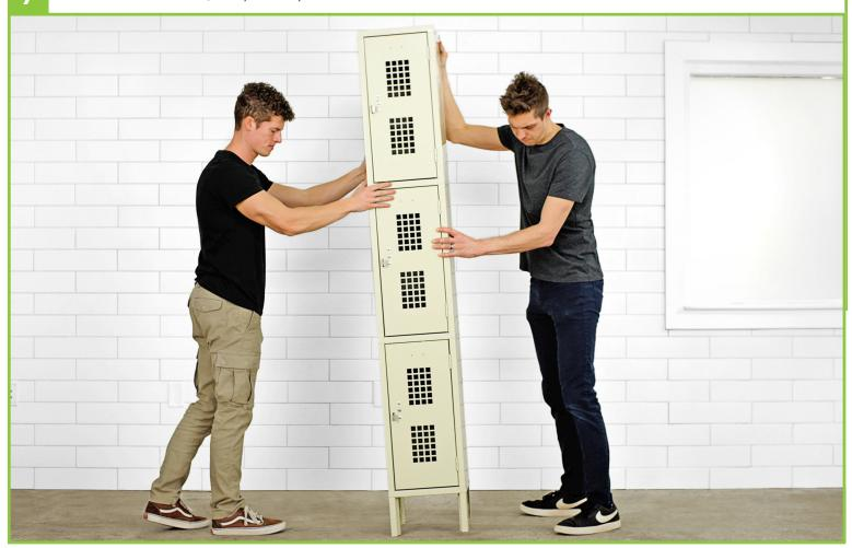
Inspect the outside of the locker – front, back, and sides. Finish bolting any shelves, side panels, back panels, and extension legs, ensuring that all pieces are bolted together. Tighten bolts with ratchet if necessary.
