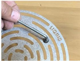
**Step 2.** Unscrew the nut on grate
