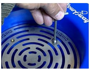
**Step 3.** Align screw in hole and tighten with tool
