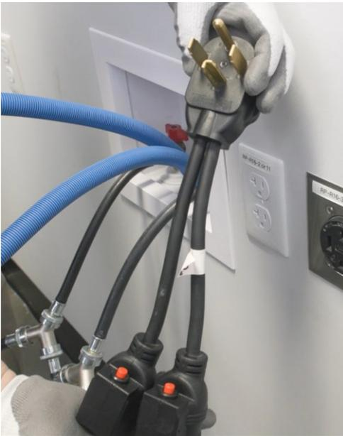
1. Confirm that your 240V outlet is functioning properly and is compatible with a 4 prong NEMA plug.
