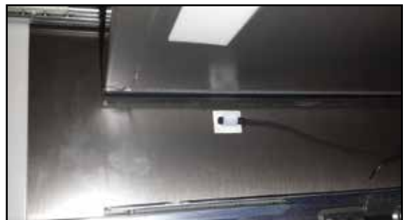
Figure 7-3.6. Refrigerator Meat/Fish Bin Temperature Probe
