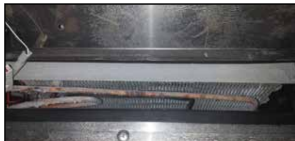
Figure 6-11. Evaporator Coil
