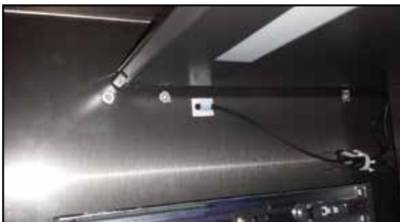
Figure 7-3.5. Refrigerator Deli Bin Temperature Probe
