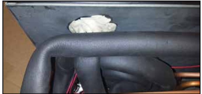
Figure 6-1.1. Sealing Compound (Inside)
