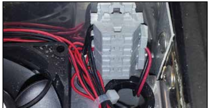
Figure 6-14.2. Evaporator Terminal Block
