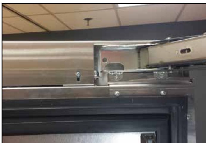
Figure 7-4. Door Magnet (Reed Switch)
