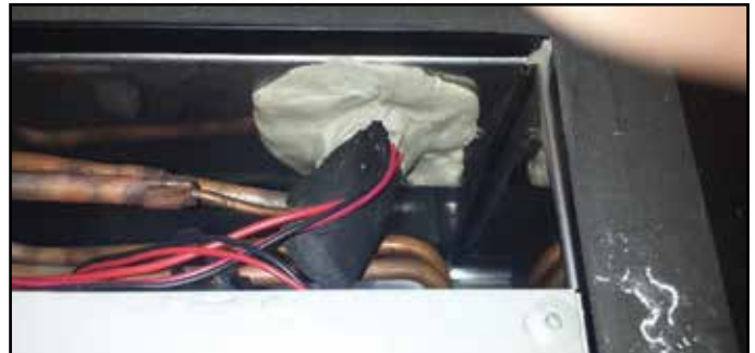
Figure 6-1.2. Sealing Compound (Outside)
