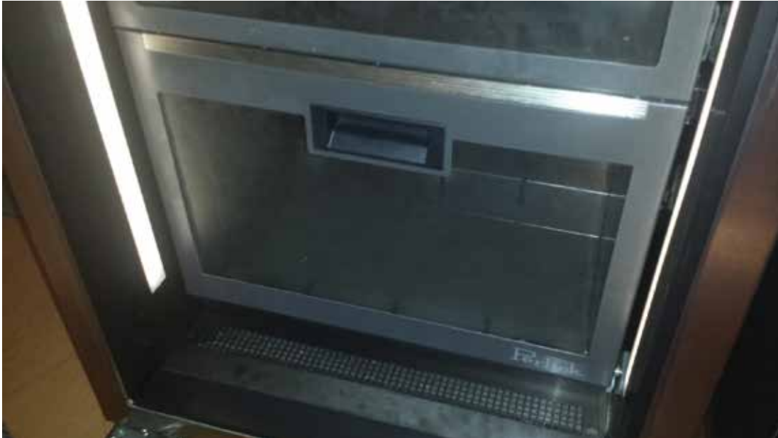
Figure 9-8. Damper Tip-Out Bin
