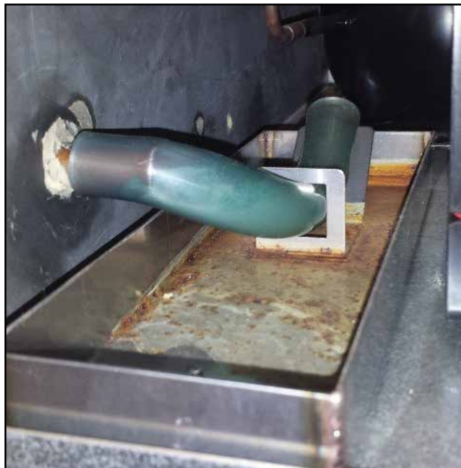
Figure 6-3. Evaporator Condensate Drain
