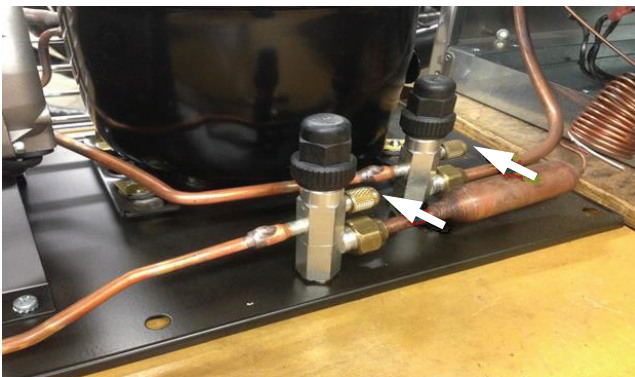
Figure 6-7. Service Valves
