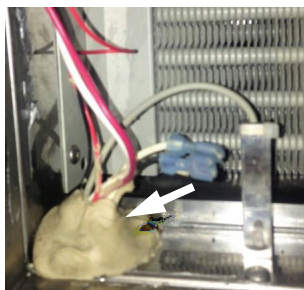
Figure 6-1. Sealing Compound at Wiring Pass-through
