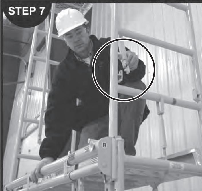
Attach the bottom of the braces at the bottom of the extension ladders.
