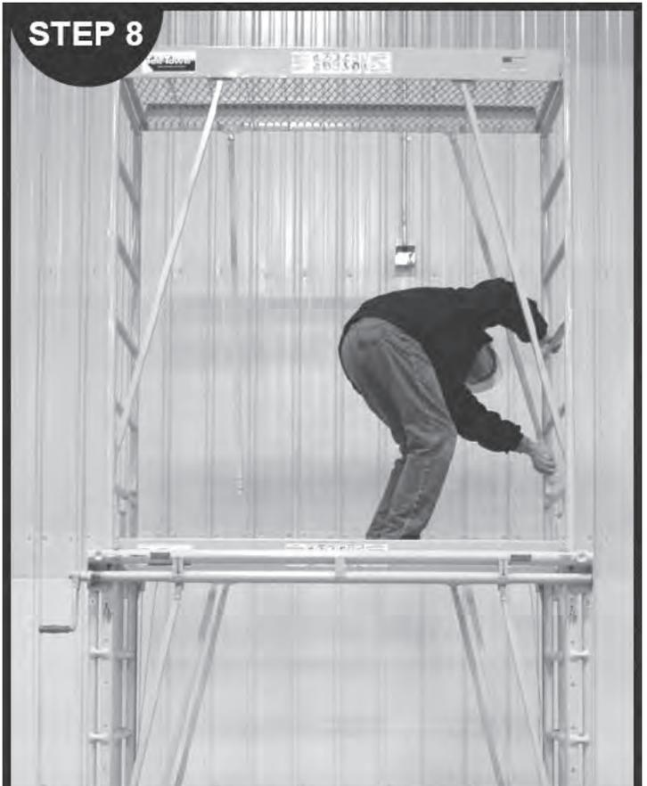
Attach all four braces before using.
