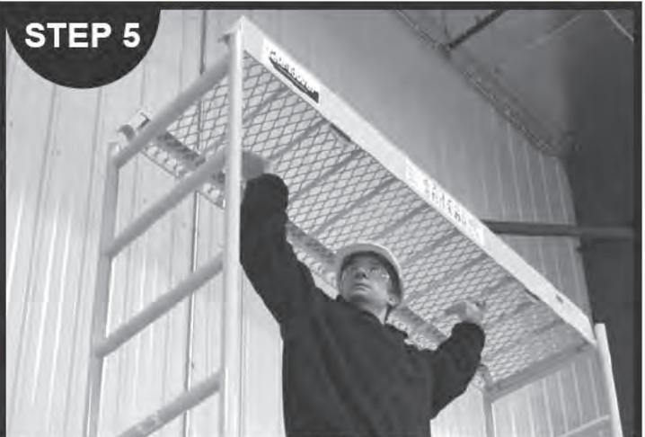
Position deck on the **TOP RUNGS** of the extension ladders only. **NEVER** position the deck on any of the lower rungs as this will prevent proper installation of the anti-sway braces resulting in an unstable structure.
