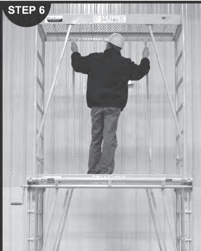
Attach the braces to the bottom of the extension deck.
