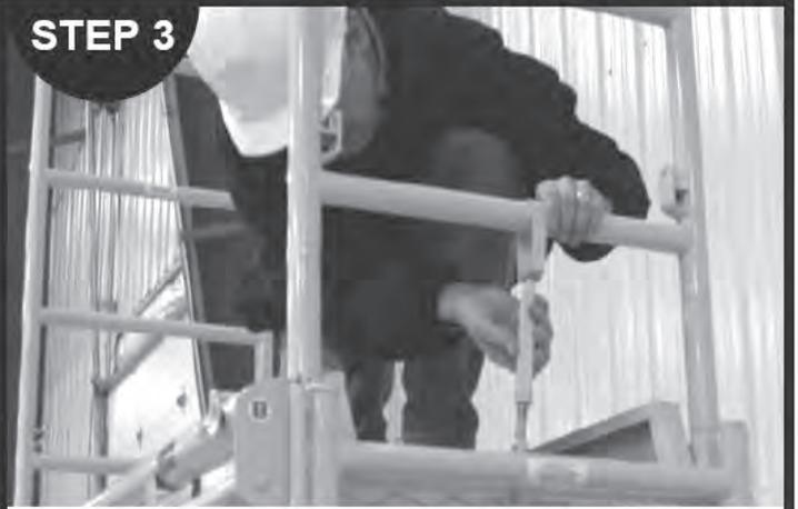
Loosen the turnbuckles on the extension ladders and turn them down toward the deck.
