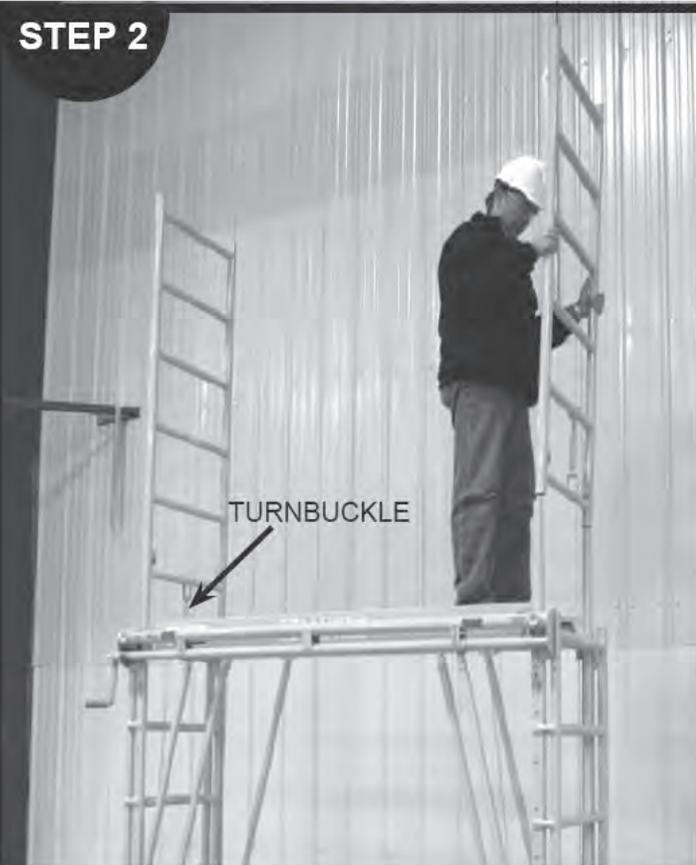
Place the extension ladders on the coupler pipes with the turnbuckle fastener on the bottom as shown.
