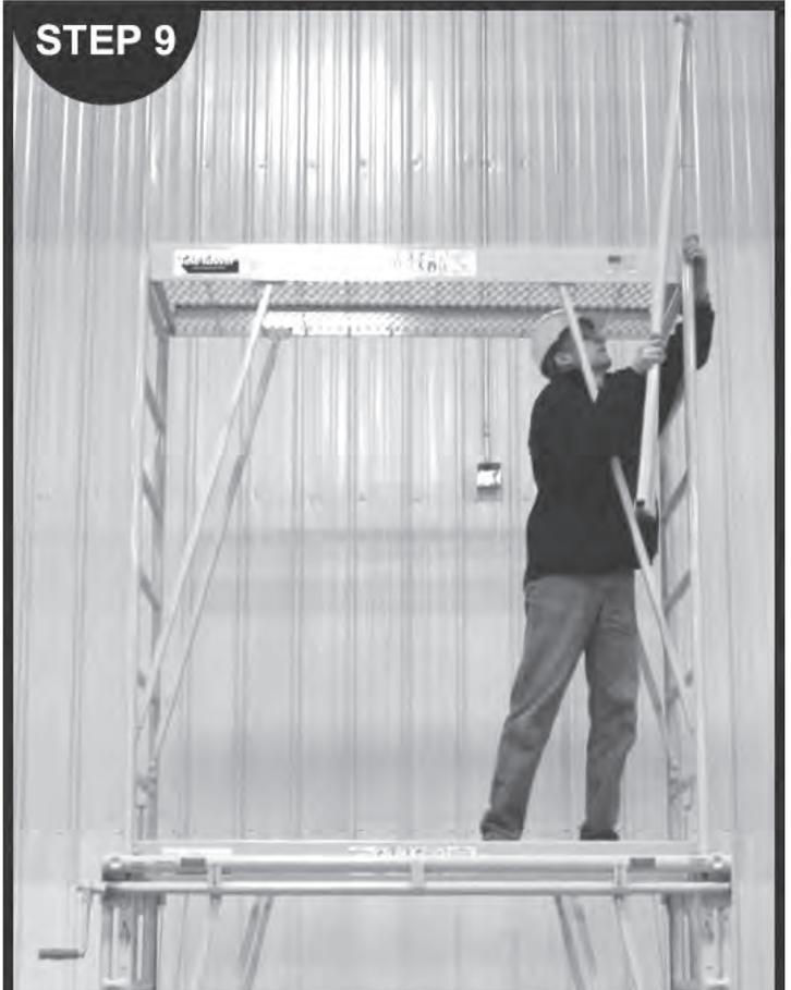
Insert the safety rails in the top of the extension ladders.
