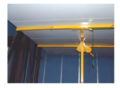
Assemble the cab walls under the ceiling.
