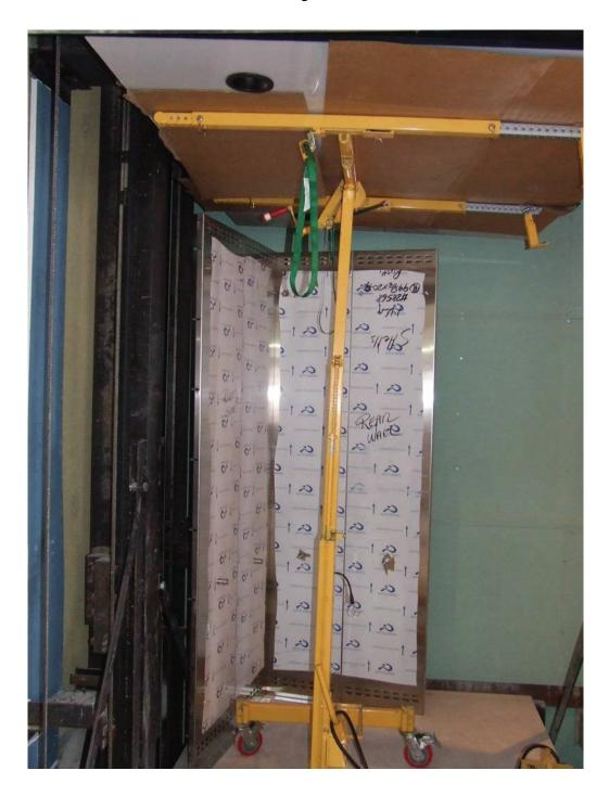
Note: Be careful not ot hit or damage the ceiling when assembling the cab walls.
