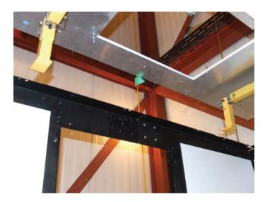
Open the emergency ext and access the canopy from a ladder. Using an alignment tool, insert the tool through a hole in the canopy and into a hole in the back wall to secure the back wall while installing the hardware in the canopy.
