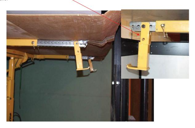
Remove the pendant station and stand outside the hoistway when lifting the ceiling.
