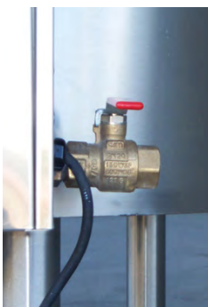
2. Turn off the manual gas valve at the rear of the unit.
