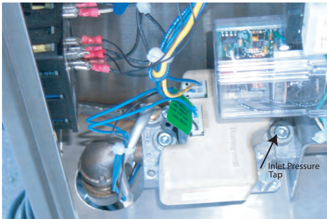
Fig. 1.4 Inlet Pressure Tap
