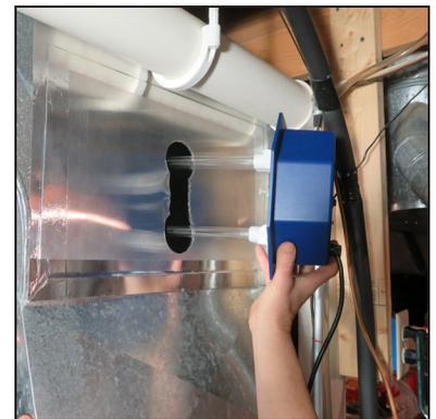
9. Attach the system to duct work with the 8 sheet metal screws using a 1/4" nut driver. Make sure to tighten screws evenly.
