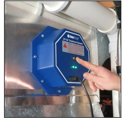
14. After 24 hours, set the fan switch on the thermostat into "AUTO" mode. The system is now operational and will only turn on when air flow is detected.
