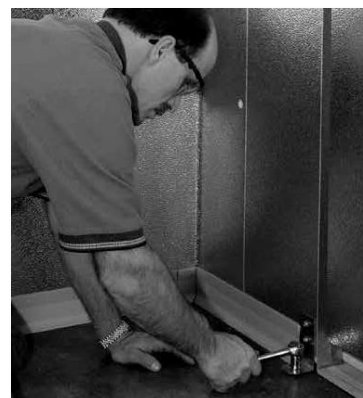
Attach slam brace with fastener provided
