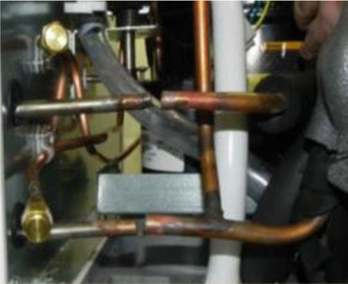
Once unit is recovered, unsolder Evaporator refrigerant lines
