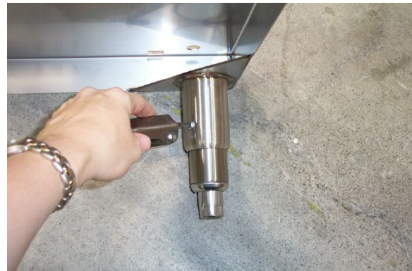
Figure 2—Tightening the legs
