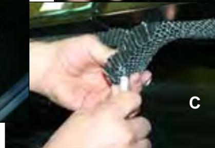
View of Honeycomb Air Diffuser (Typical on All Cases)
