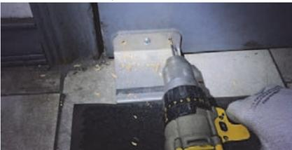
5. Remove the installation screw and flip the bracket over so the grip tape surface faces up.
