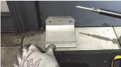
3. Drill through the center hole with a 5/32" drill bit to a depth of 1 1/4" and then insert and tighten one of the provided sheet metal screws.
