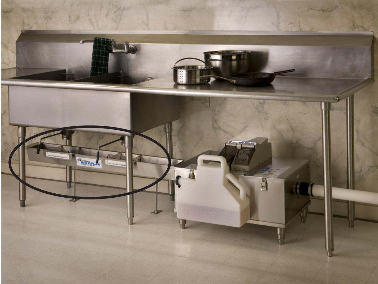
**A HAG-2 Horizontal Air Gap Assembly coupled to a Big Dipper® W-200-IS Point Source Automatic Grease Removal System. Optional HAG-BA-1 Solids Strainer Baskets are shown in this picture.**
