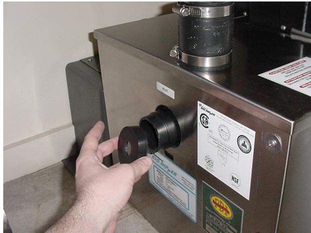
***Before Installing the HAG Horizontal Air Gap Assembly, remove the Flow Control located on the Inlet end.***
