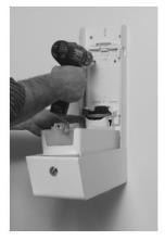
**Step 4:** Place dispenser in metal cover, lining up with 3 dispenser mounting holes inside metal cover. Secure with recommended fasteners.
