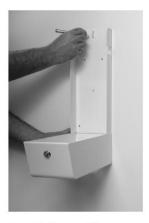
**Step 1:** Place metal cover on wall in desired location. Make sure metal cover is straight and level. Using the metal cover as a template, mark the 4 metal cover mounting holes around the outer edge of the cover. Mark the 3 dispenser mounting holes on the wall.
