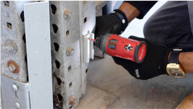
STEP 1. Install the mounting extrusion in the lowest rack insert from the ground.
