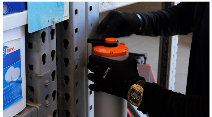
STEP 6. Straighten the canister so it is parallel with the wall. Then, install the 2nd plastic bracket so it slides into the top of the canister.
