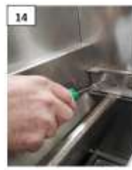
14 BURNER CONNECTING SHEET SCREWS ARE INSTALLED
