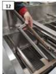
12 THE BURNER IS REPLACED
