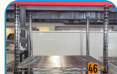
**D** Install the wire rack shelf designated for box storage at Slot #46.
