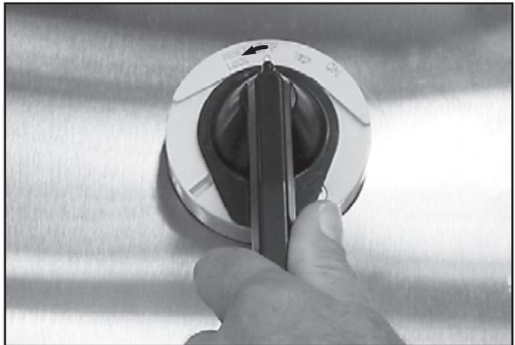
3. Engage the handle lock and insert a locking device to prevent the Breaker Switch from turning. Attach a tag on the Breaker Switch to indicate that work is being performed on the circuit.
