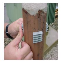
Step One – Install 2 or 4 self-adhesive Gripper Tabs around the top of the bollard with "fingers" pointing down, and 2 or 4 more near the base of the bollard. If there is a small space to fill between the bollard and the cover, use 2 Gripper tabs evenly spaced around the bollard. To fill a larger space, use four Gripper Tabs at the top and bottom.
