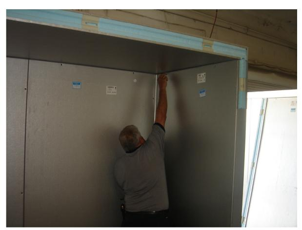
7- Begin at one end of the walk-in, positioning roof panels, locking them to adjacent wall panels, and continue assembling in "rings."
