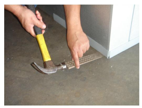
6-Install shims under vinyl screed corners and across as needed to ensure support panel joints and levelness of panel.
