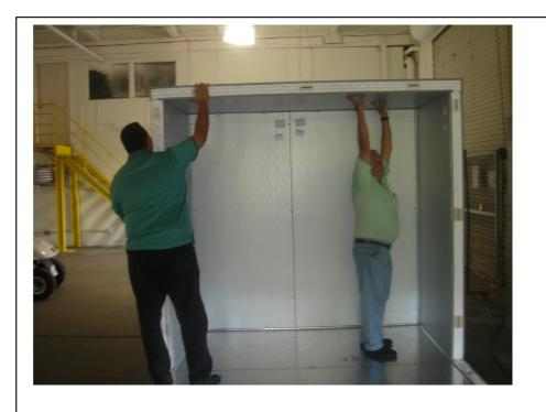
6- Finish corner by installing ceiling panel, and continue assembling in corresponding floor/ walls/ ceiling in "rings."
