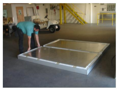
1— Set the floor Panels according to the setup Drawing.
