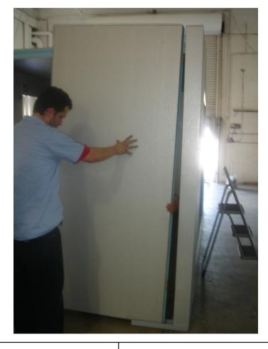
3-Seal with silicone both the inside and the outside edges of the wall panels
