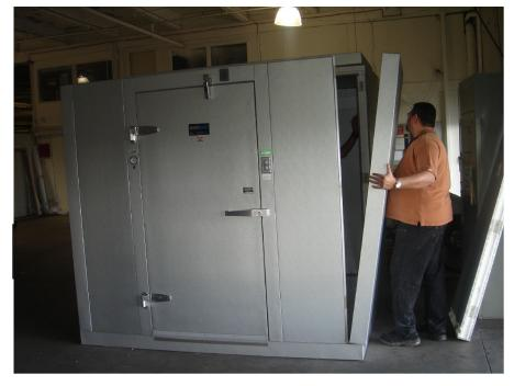
4- Begin with two Corner Panels and secure to Floor panels to start making a corner. Make sure that the top of each wall panel is flush with each other.
