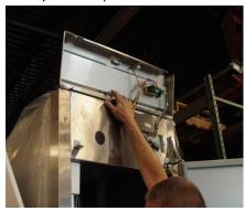
4) Remove the Phillips screw from the top & bottom hinge
