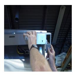
13) Put the top panel of the unit back down to its proper position and install the screws back into the panel.
