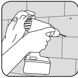
2. Drill holes for screw anchors.
