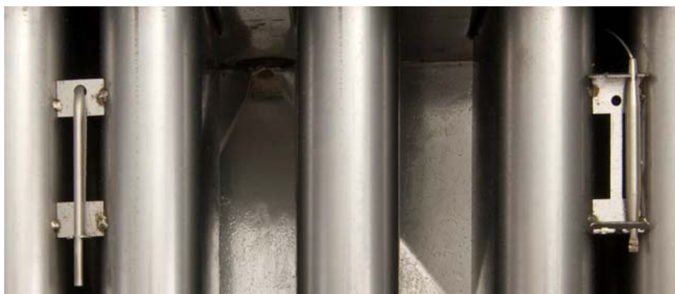
Typical sensor probe/high-limit locations and mounting hardware.
