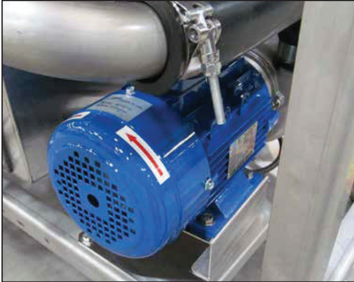
Fig. 23 - Motors rotate counter-clockwise.
