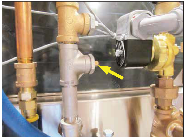
Fig. 21 - Rinse-aid injection point.
