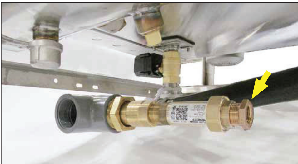
Fig. 6 - Mechanical DWT valve.
