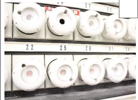
3. If you have External Circuit Fuses. Check and replace broken Fuses
