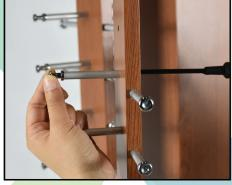
Insert end cap and tighten screw.
