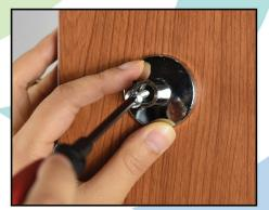
Fix support base to top and bottom of square wood pipe. Use 1" screw (x8) in total.
