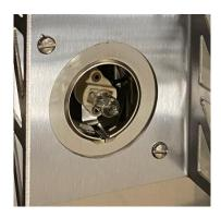
8. Then replace the light gaskets with new gaskets onto the light globes and reinstall them onto the light fixtures.
