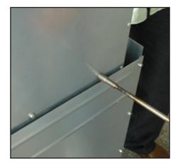
3. Slide the flue wrap over the flue.
