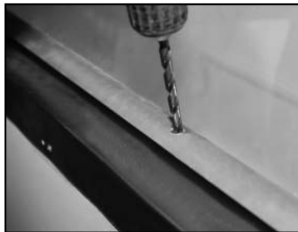
Image 3 (Drilling lock bracket hole)
