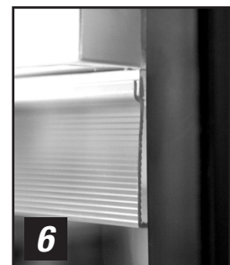
6 lampshield "U" channel in position over metal bracket.
