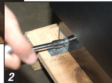
2 Removing bracket from cabinet.
