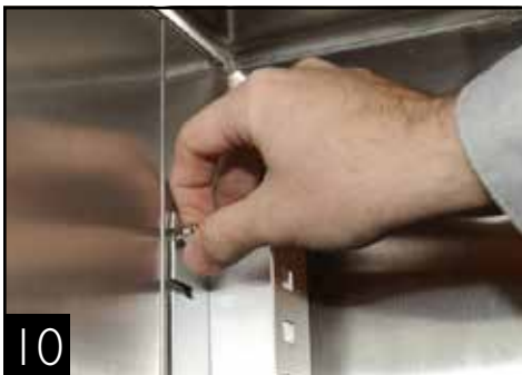
Pilaster installation (side wall of cabinet)
