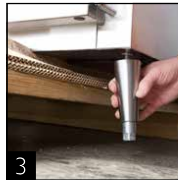
Thread leg into cabinet bottom cabinet.
