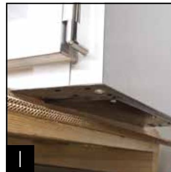
Slide packing material under the unit.
