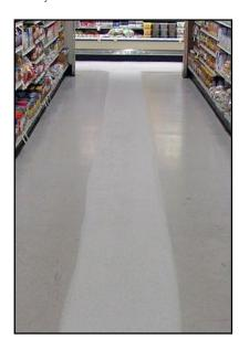
One pass with an orbital scrubber equipped with a surface prep pad
