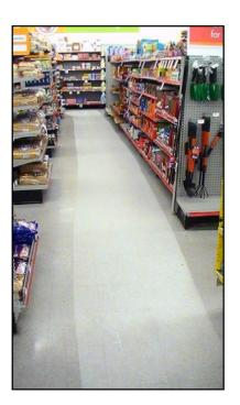
Finish removed with a 20-inch orbital scrubber using a surface prep pad
