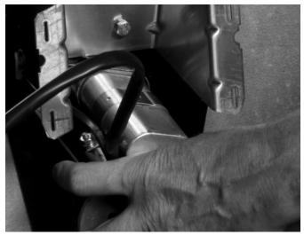
5. Grasp the gearmotor as the second pin is removed. Pivot the gearmotor out of place.
